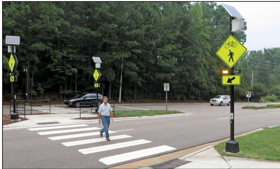
Figure 15- Crossing equipped with Rapid Flash Beacons
