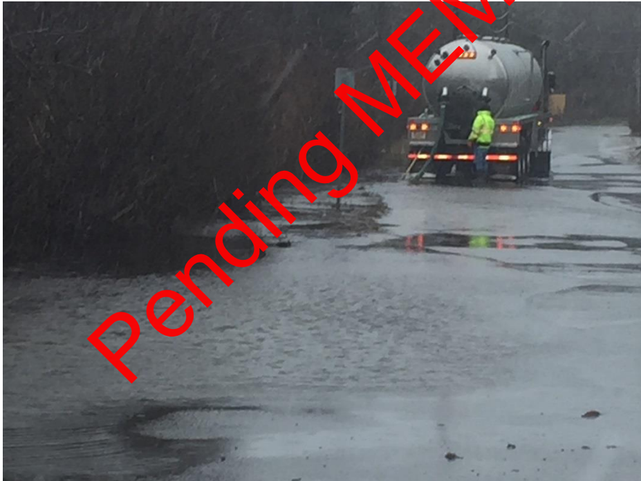
Road under water.
