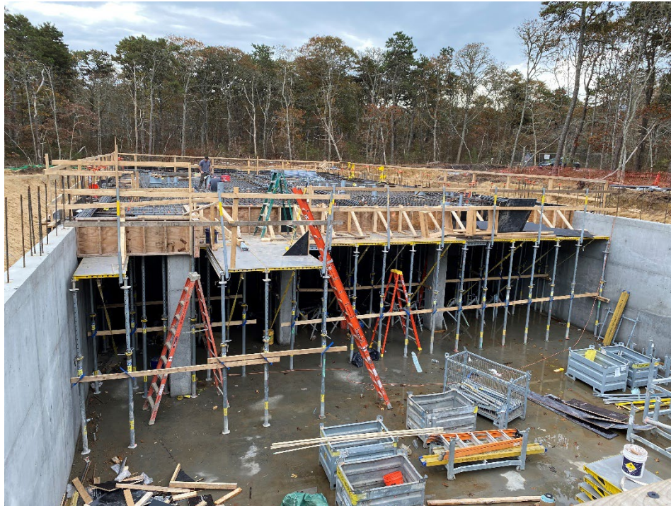
First Floor Slab Formwork at Wells 5 & 8 PFAS Water Treatment Site
