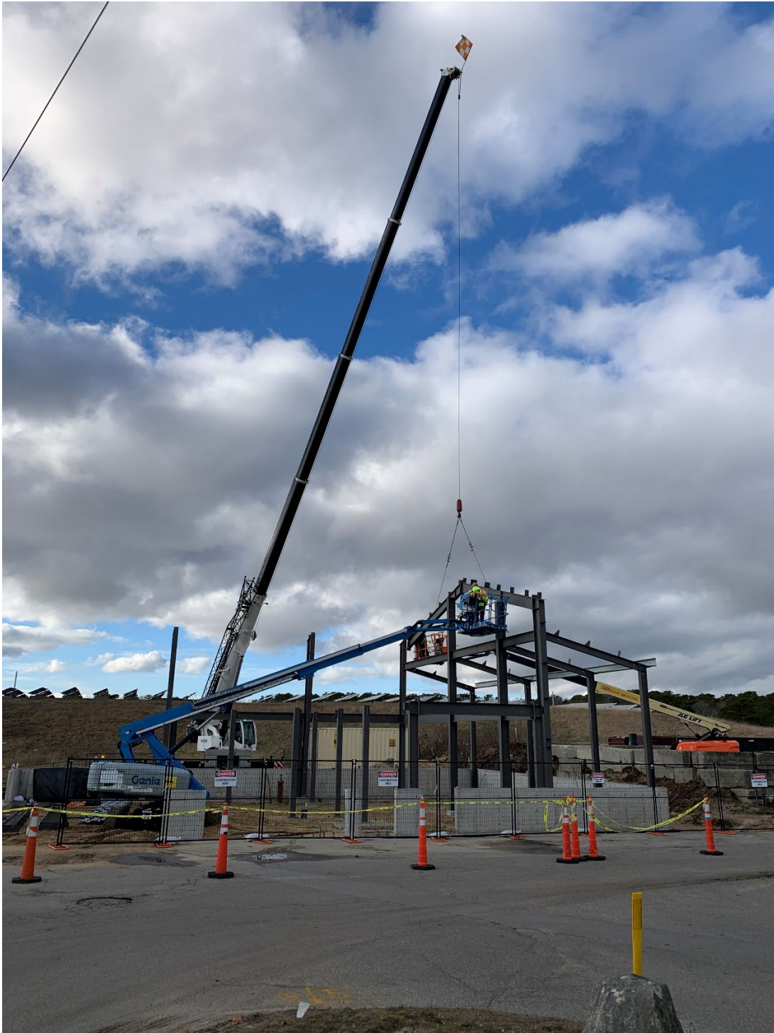
Steel Erection work at Transfer Station – Phase II (Priority I)
