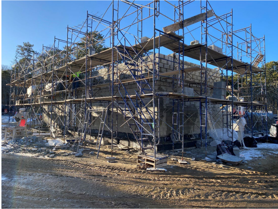
Wells 5 & 8 Treatment Plant – Wall Construction
