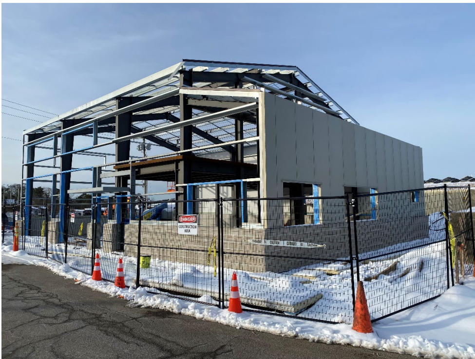
Insulated Panel Installation at Transfer Station – Phase II (Priority I)
