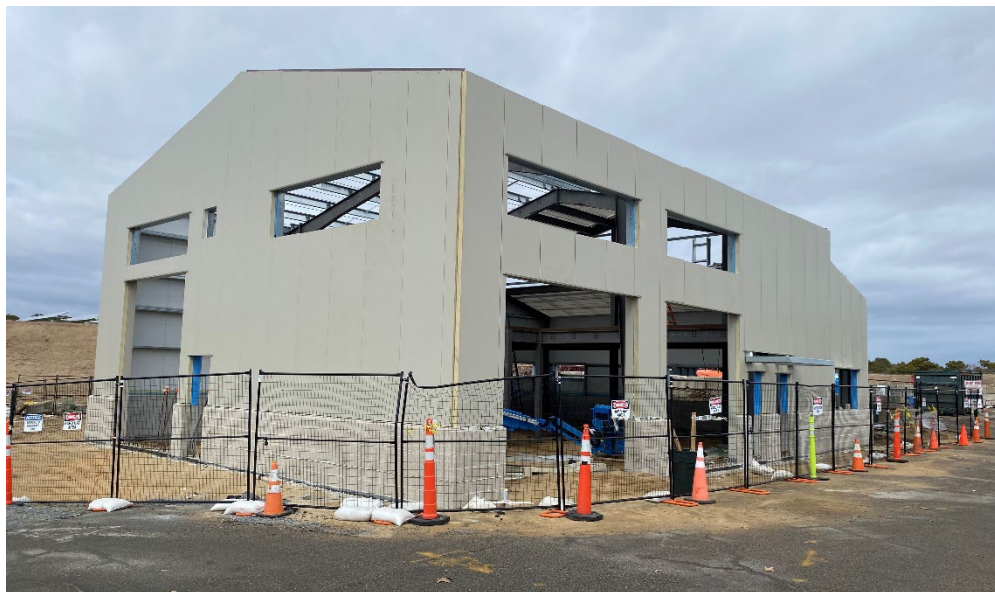
Insulated Panel Installation at Transfer Station – Phase II (Priority I)
