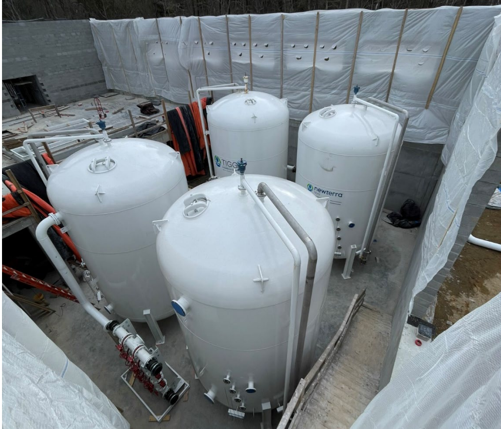
Wells 5 & 8 Treatment Plant – Wall Construction
