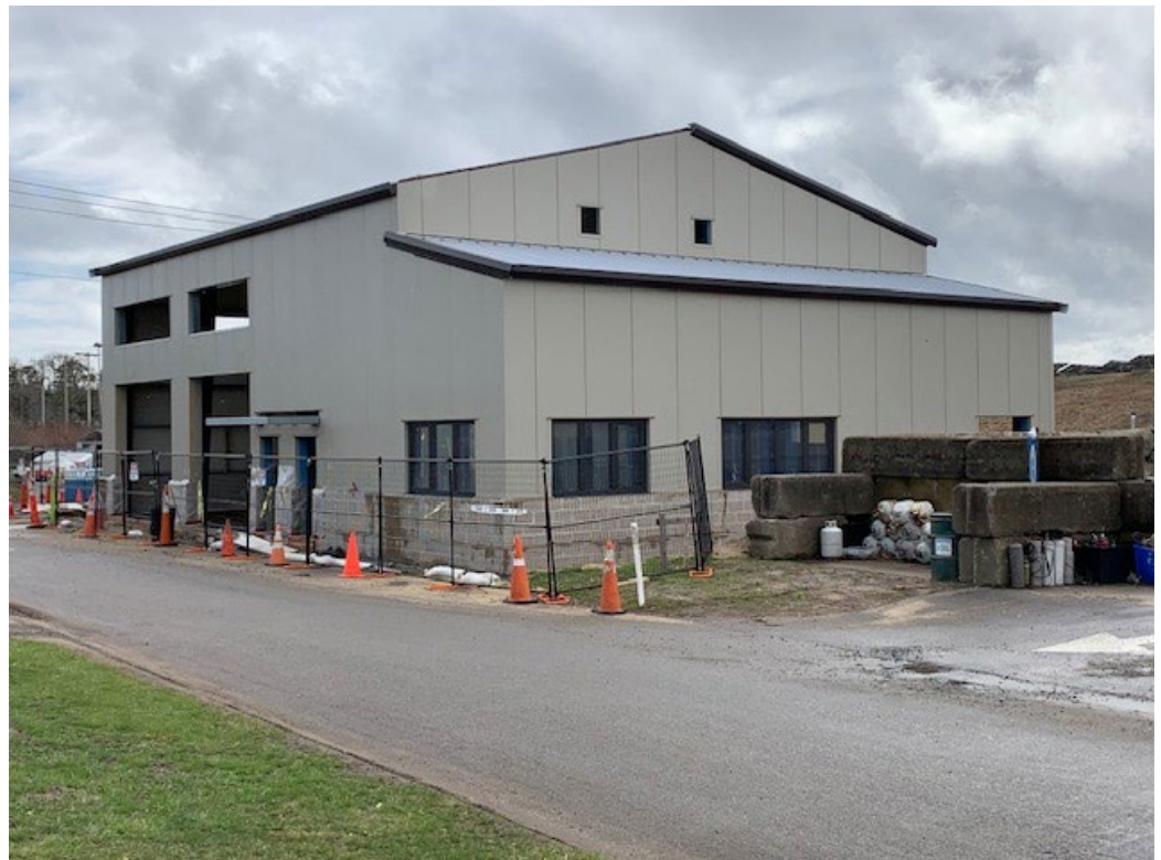
Building Envelope Construction at Transfer Station – Phase II (Priority I)
